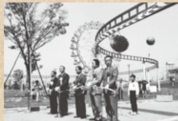
堀内公園完成 Horiuchi Park is completed
